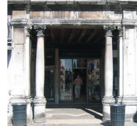
Clock Tower renovation by Tomaso Temmanza. The two interior columns were added and a crack now appears above each. FOTO BY AUTHOR
