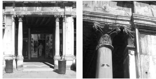
Figure Two: Clock Tower renovation by Tomaso Temmanza. The two interior columns were added and a crack now appears above each. Photo by author.
